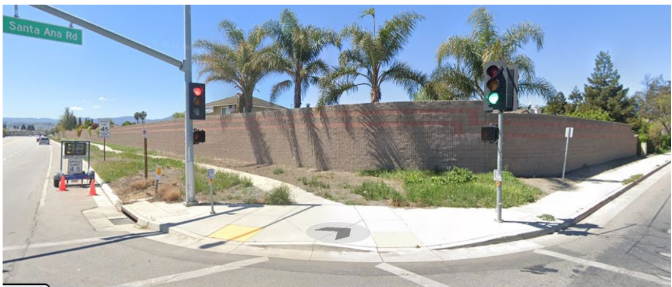
Figure 1 Corner of Santa Ana & Highway 25, facing southwest
