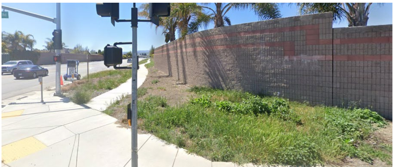
Figure 2 Corner of Santa Ana & Highway 25, facing southwest
