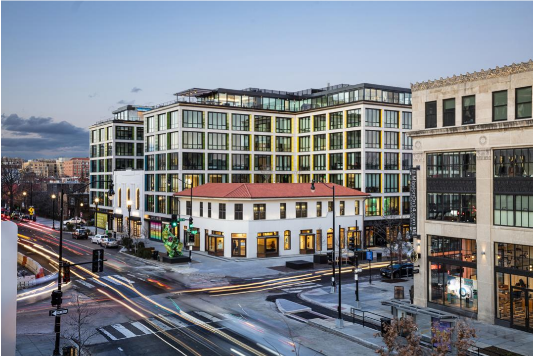
View of site looking northeast. New sculpture will be installed where “Material (SG) I,” a sculpture on loan from Yinka Shonibare, was formerly located.
