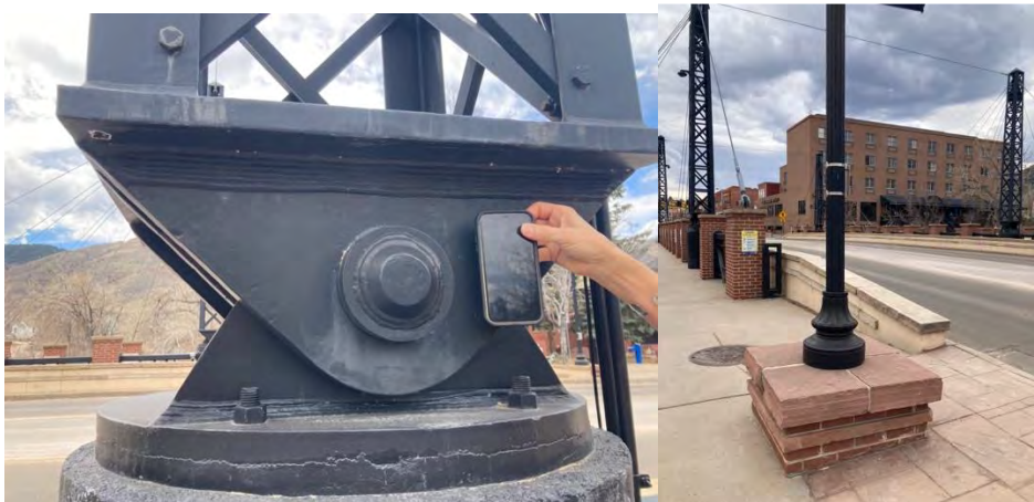
Location #6: Northeast structural support on Washington bridge
