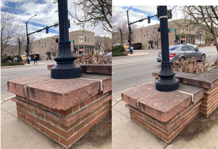
Location #3: South Light Pole at 10 th and Washington
