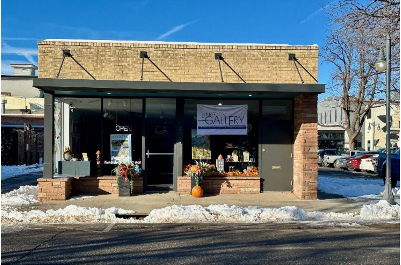
East Facade – Building Entrance
