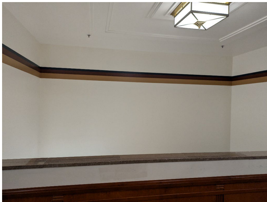
Top of stairwell facing south
