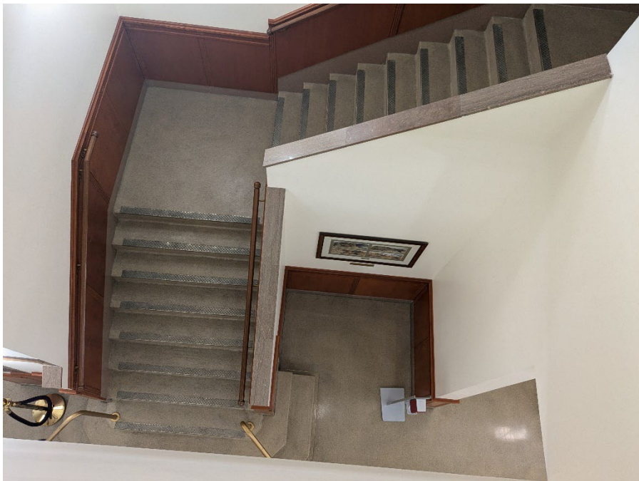
Looking into stairwell from third floor to second floor
