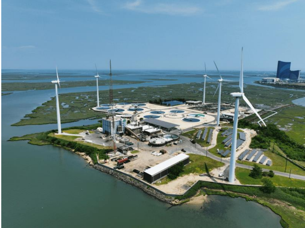
ACUA Wastewater Treatment Facility in Atlantic City.
