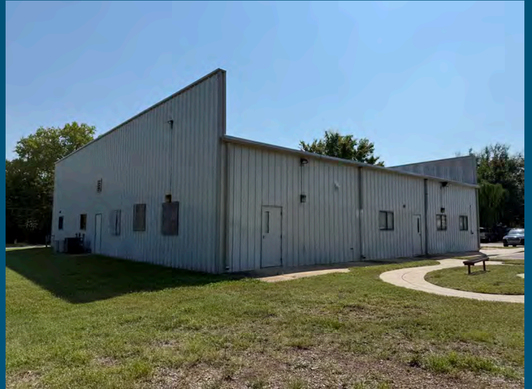
North Façade – facing basketball court Dimensions: 250' x 25'
