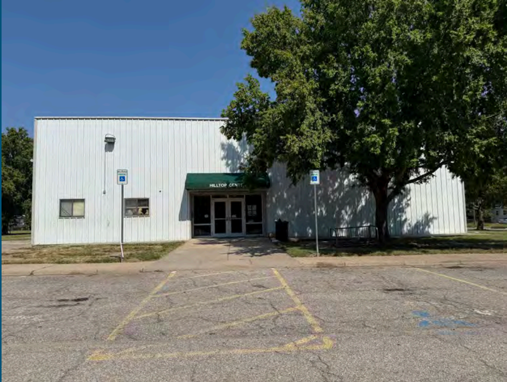
Front Façade – facing parking lot Dimensions: 250' x 25'
