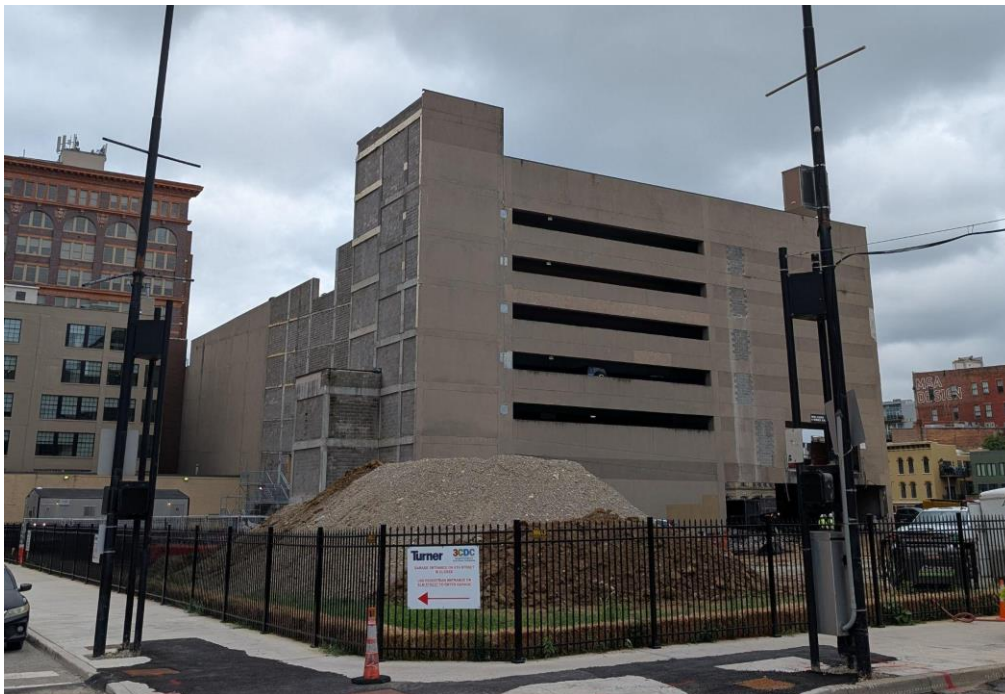
Current Garage Condition - Fall 2025
