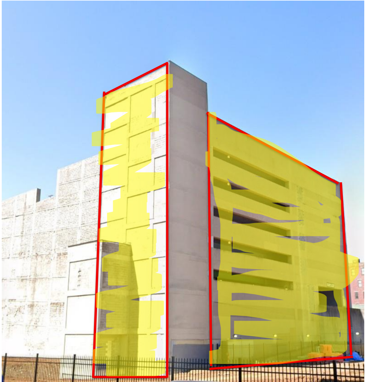
Current Garage Condition - Mural area outlined & highlighted – design to have the opportunity to wrap around the building, if desired; blank vertical section to be demolished
