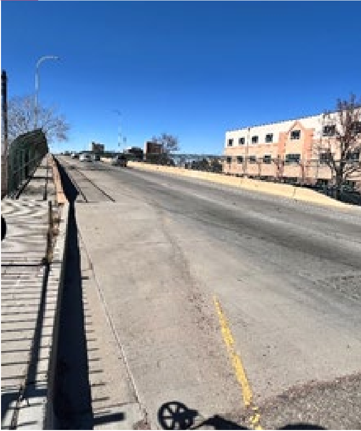
A SE corner of Lead Ave Bridge
