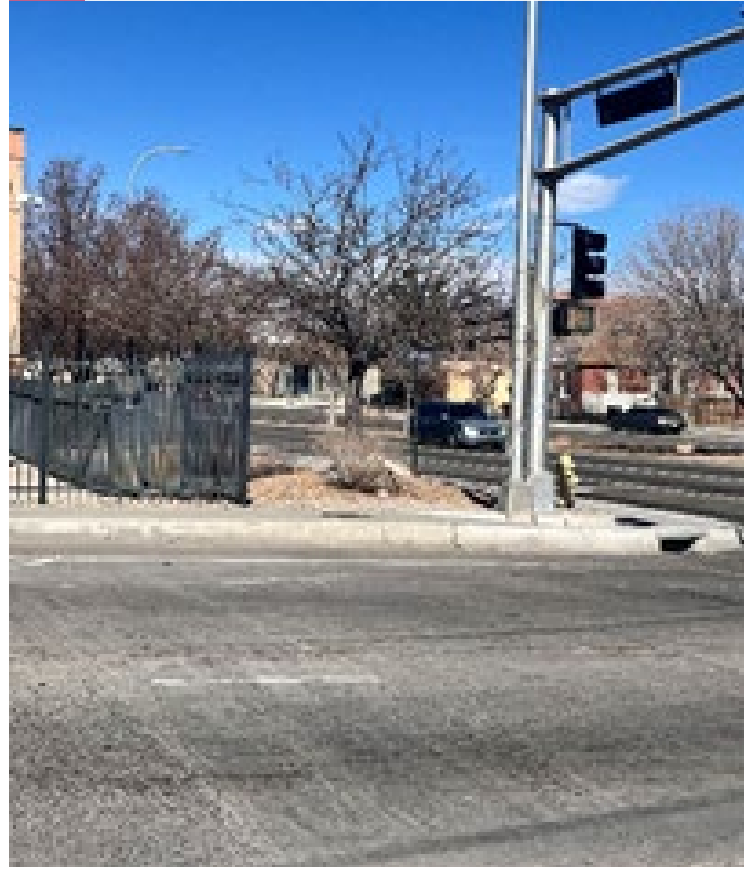
B NE corner of Lead Ave Bridge
