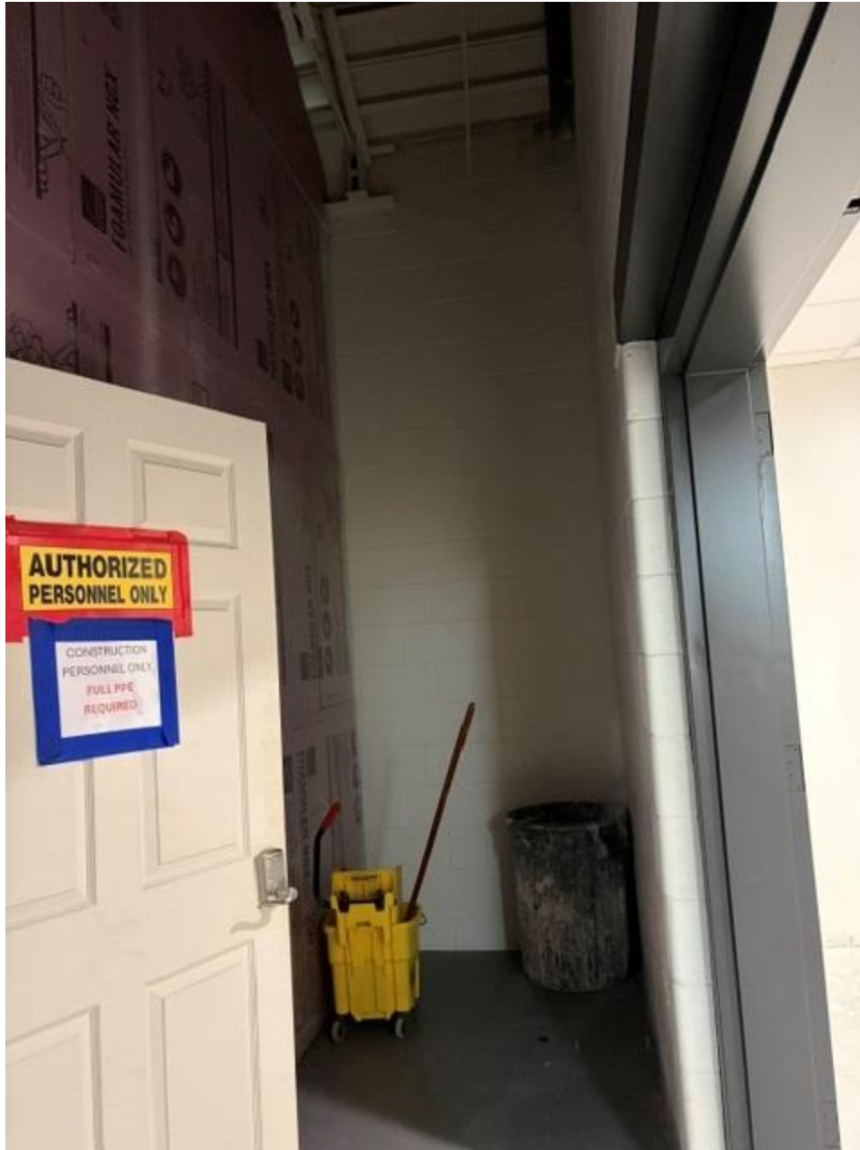
Inside the construction wall on the far right side of the wall.
