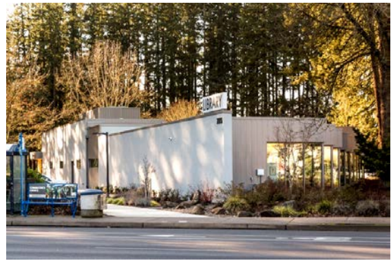
Library from street, showing reading rooms
