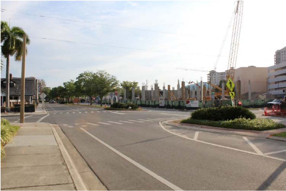
2 views from south side of intersection on Coconut Ave looking north.
