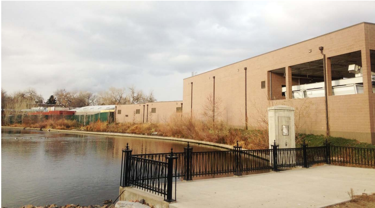
(Primary location, the Waste Management Building façade facing Duck Lake)
