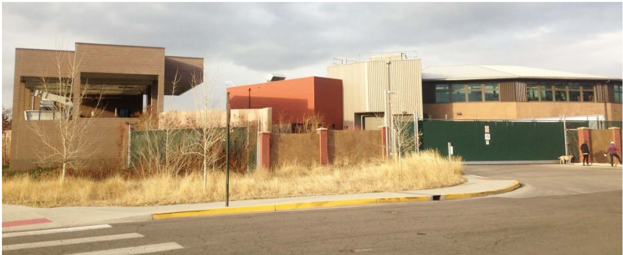
(Secondary location, fence line and service gate)
