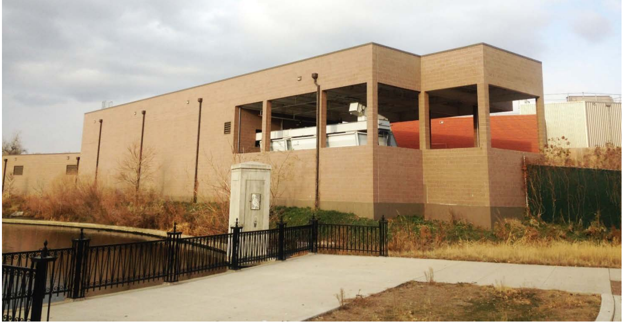
(Primary location, the Waste Management Building façade facing Duck Lake)
