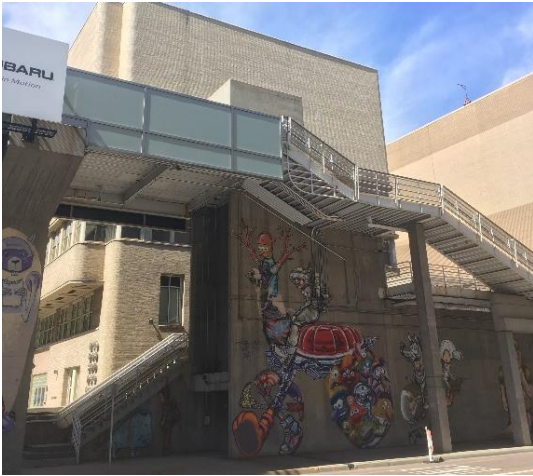
The (obscured) façade of the Commons on Champa Building. The elevator shaft and raised walkway will be removed in summer 2017.
