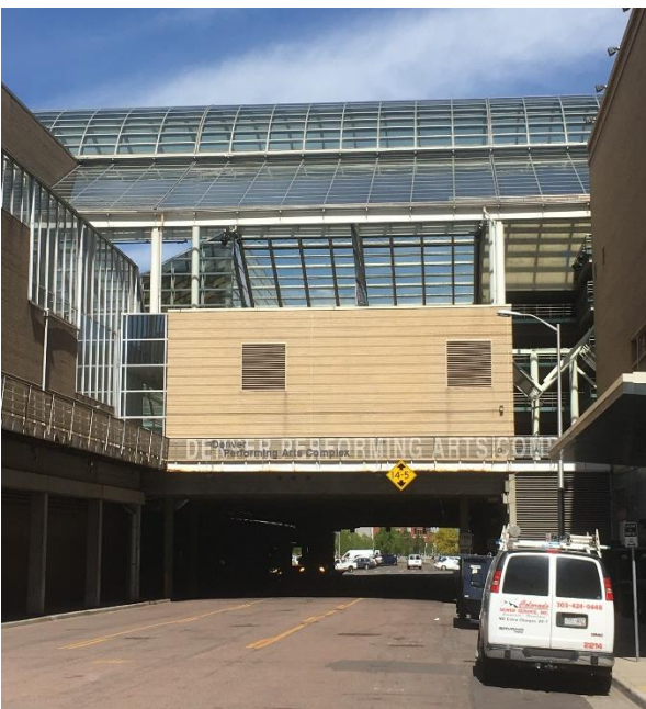
Third façade on the Boettcher Concert Hall. The raised walkway will be removed in summer 2017.
