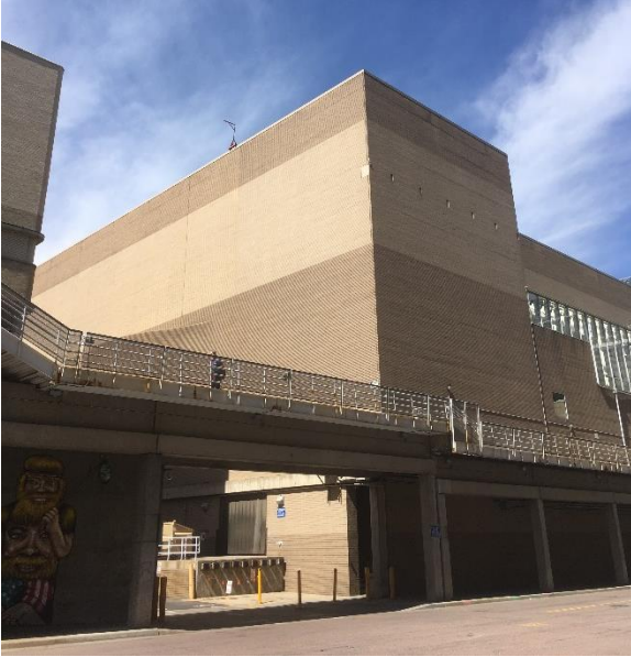
View of the two facades on the Boettcher Concert Hall. The raised walkway will be removed in summer 2017.
