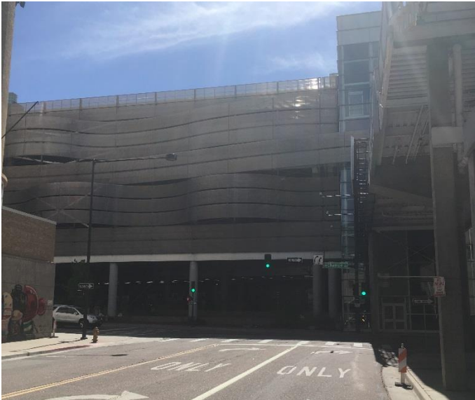
View of the Colorado Convention Center façade. The raised walkway to the right will be removed in summer 2017.
