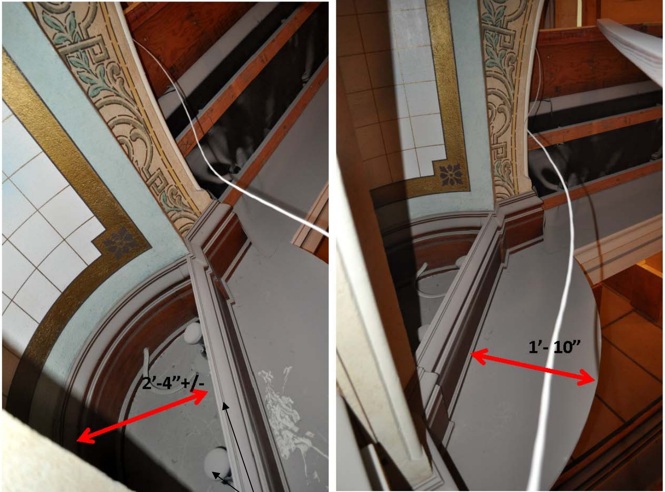
Portion of existing wood base and lighting to be removed.
