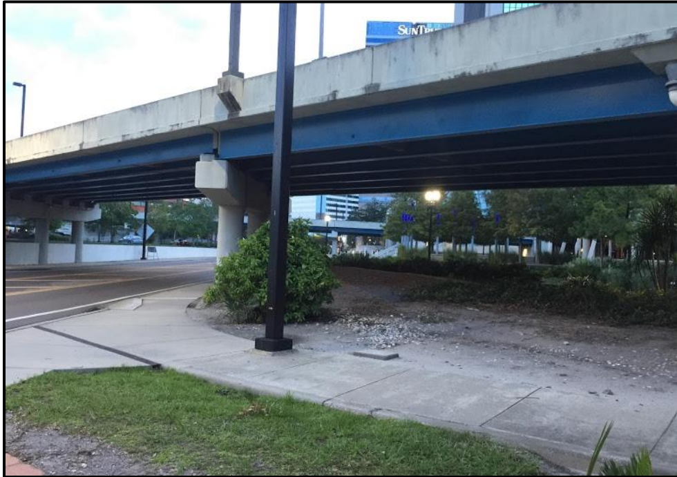
Below photo: Main Street Bridge down ramp over Independent Street
