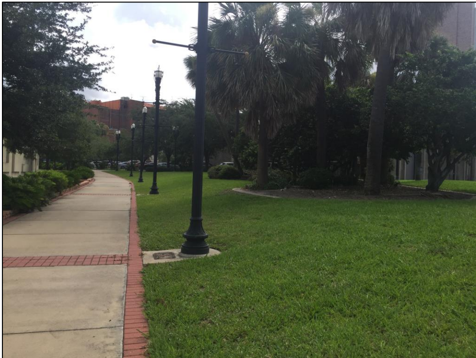
Below Photo: Sidewalk along Main Street Bridge ramp from Independent St. towards Bay St.
