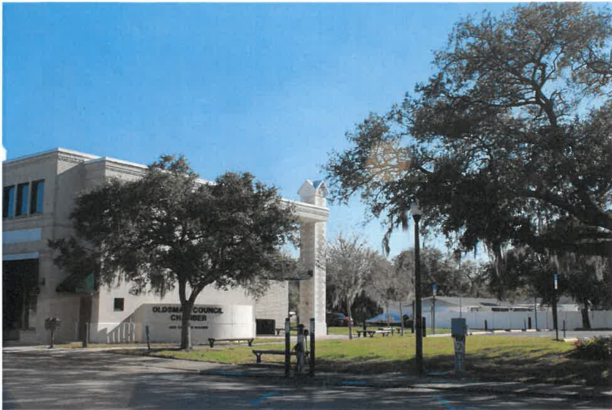
Oldsmar City Chamber, State Street, facing South East
