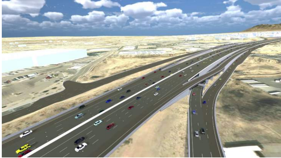
Simulation #1 – Computer generated simulation of the ultimate project. The view is looking North along the Northbound Frontage Road and Comanche On-Ramp showing the braided ramp bridge.
