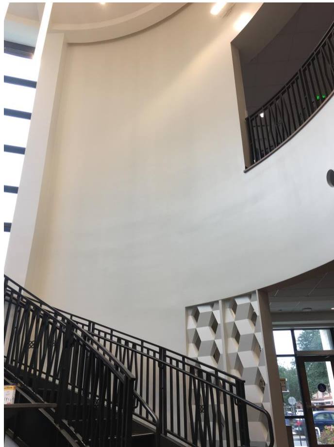
South curved wall – largest uninterrupted wall space in Beacon.
