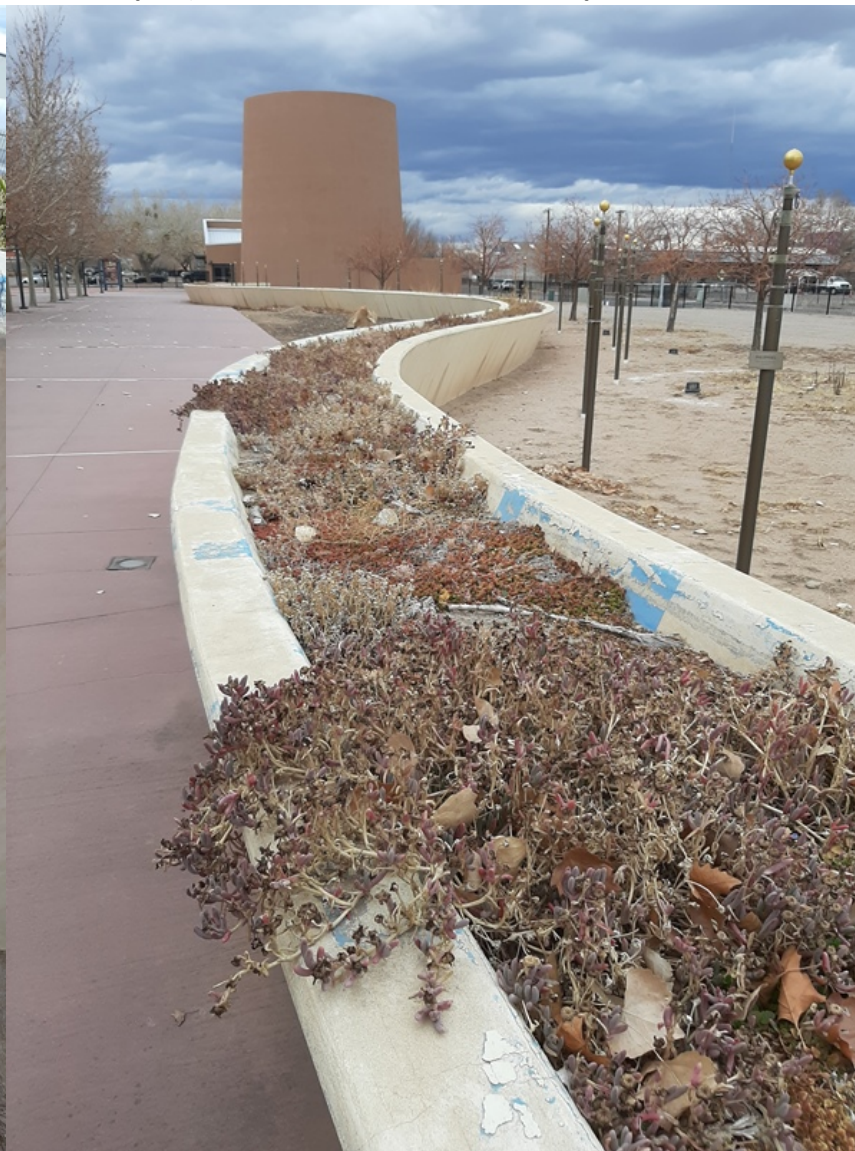
View of interior of Acequia (Interior can be considered; soil/plants can be removed)
