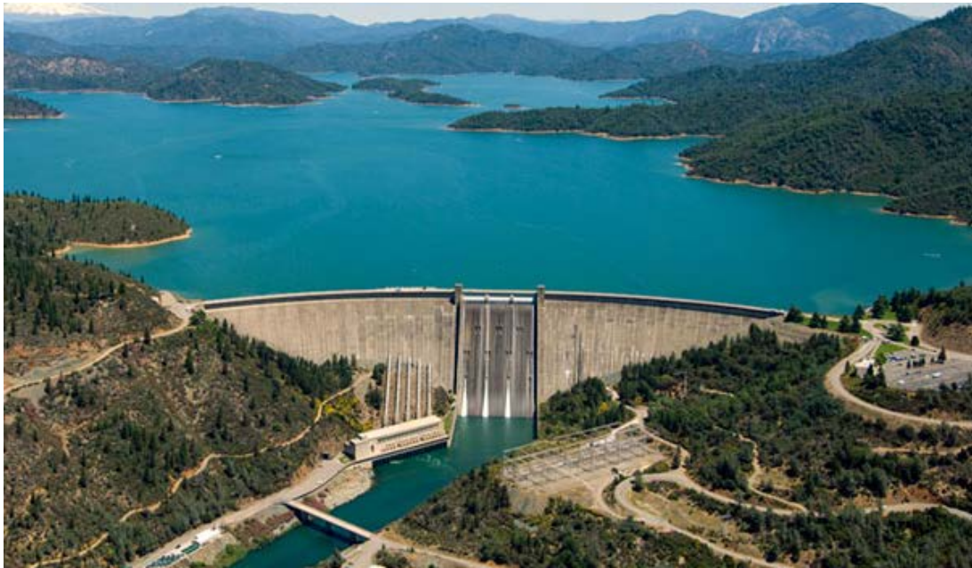
Figure 4: Shasta Dam, completed in 1945, forms Shasta Lake created for long-term water storage, flood control, hydroelectricity, and wildlife habitat. It is located ten miles upstream of the project site.
