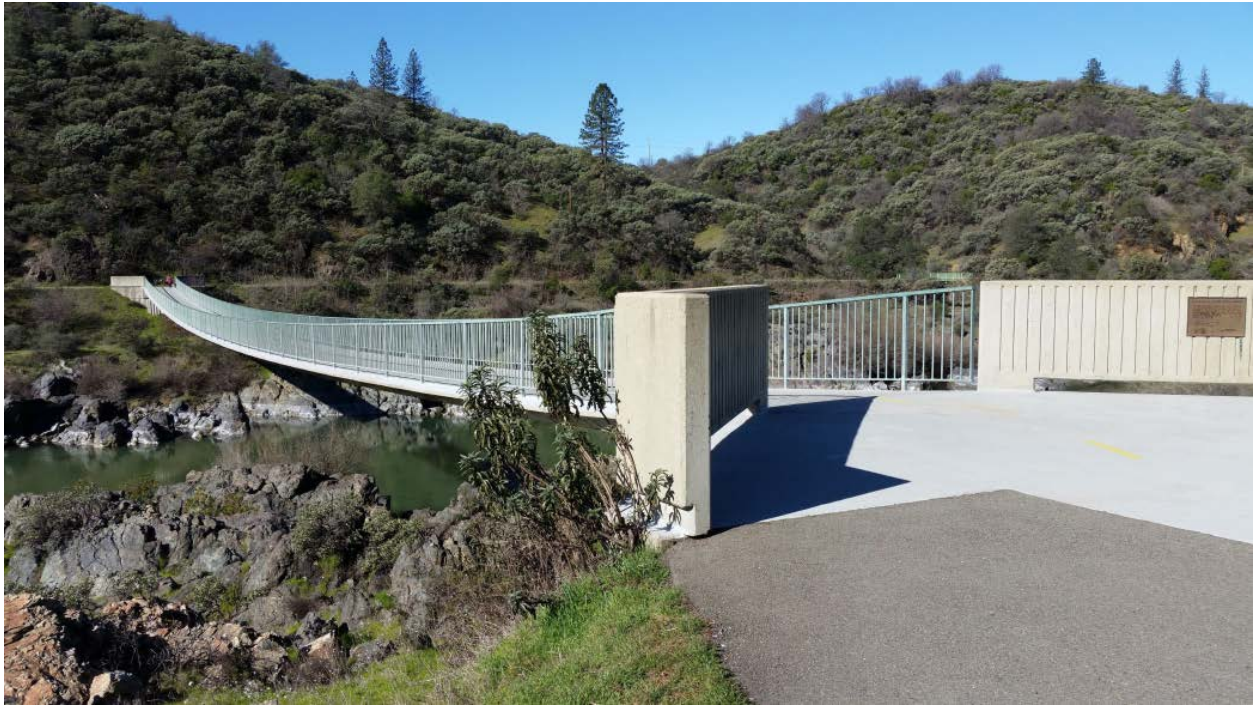
Figure 2: Photograph of the Stress Ribbon Bridge looking west
