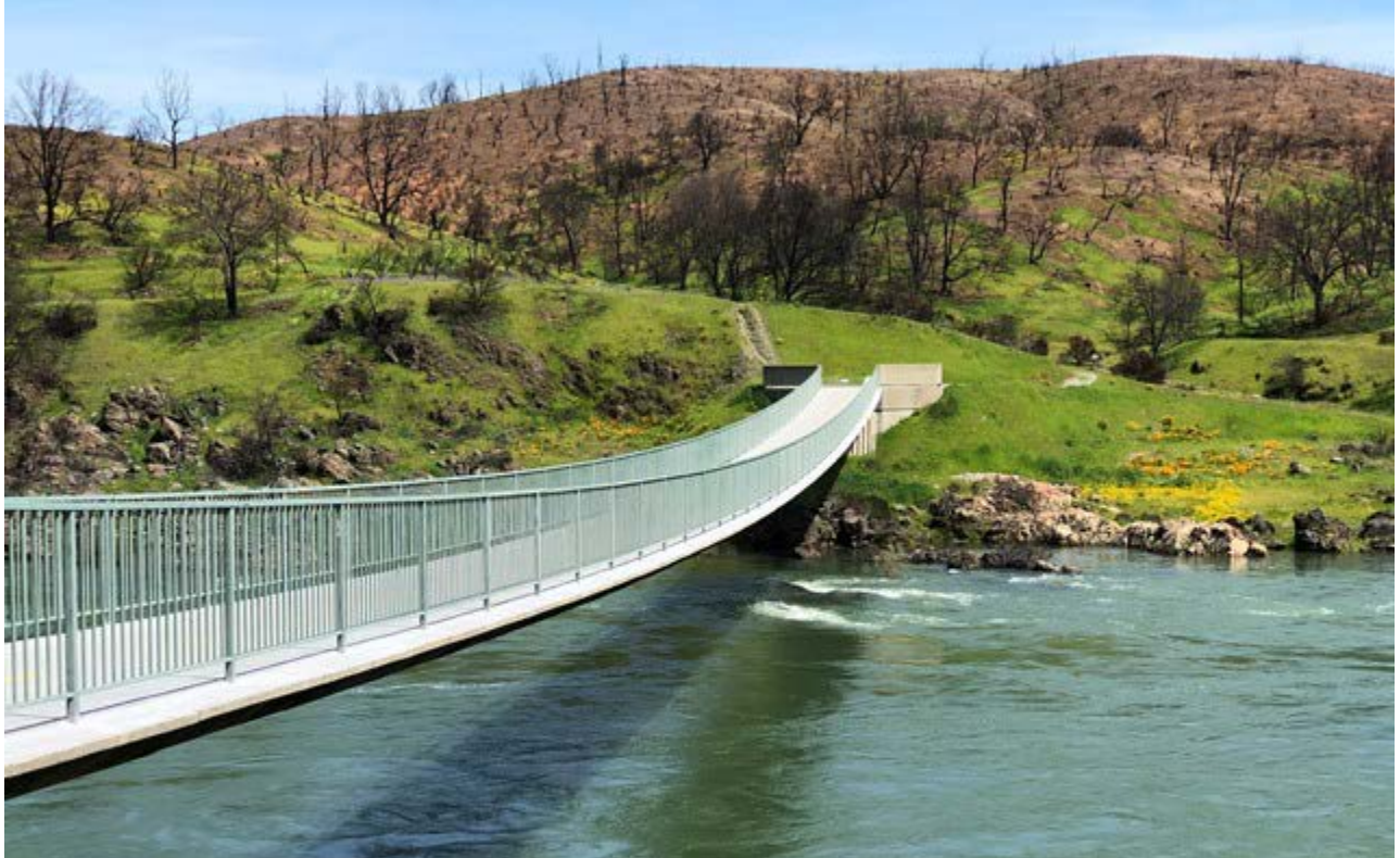
Figure 1: Photograph of the Stress Ribbon Bridge looking east
