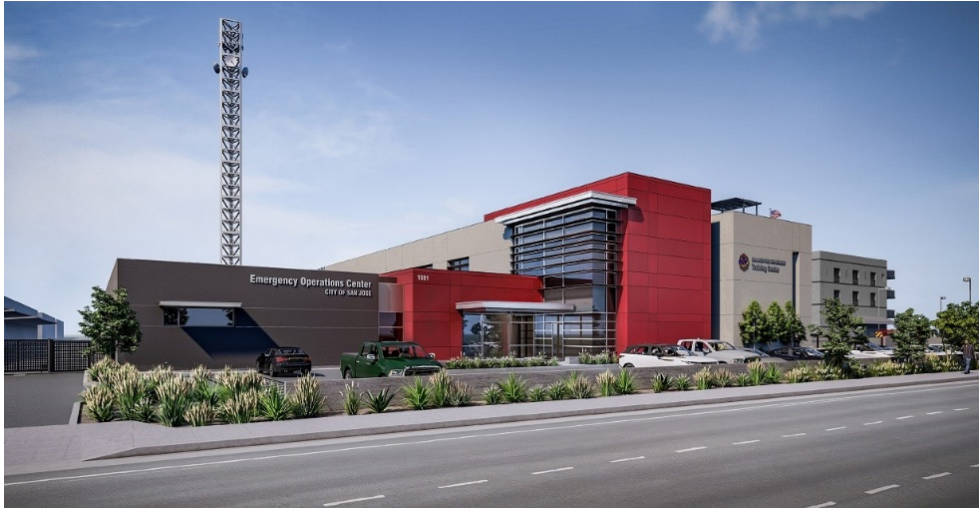
Left image: Façade of the joint facility
